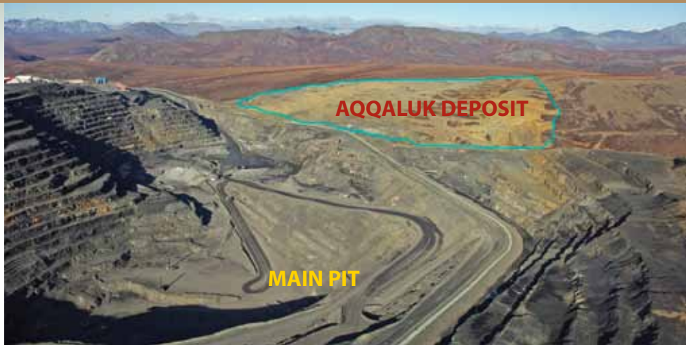
To continue operations through 2031, Red Dog needs to expand to the adjacent Aqqaluk Deposit.
