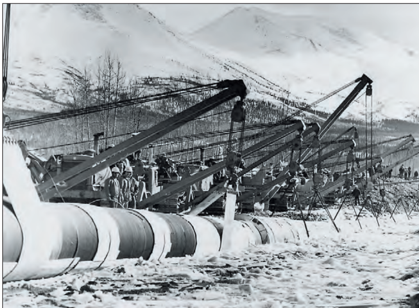
Construction crews place a segment of the pipeline into the Tonsina River in 1975. At the time construction began in 1974, TAPS was the largest private construction project in the world with an estimated price tag of $900 million. When completed in 1977, final costs were over $8 billion. Please see TAPS facts on page 4.
