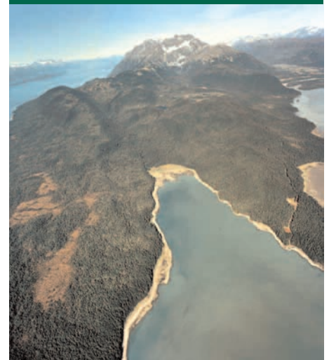
Pictured above is the port site for the proposed Kensington Mine outside Juneau.
