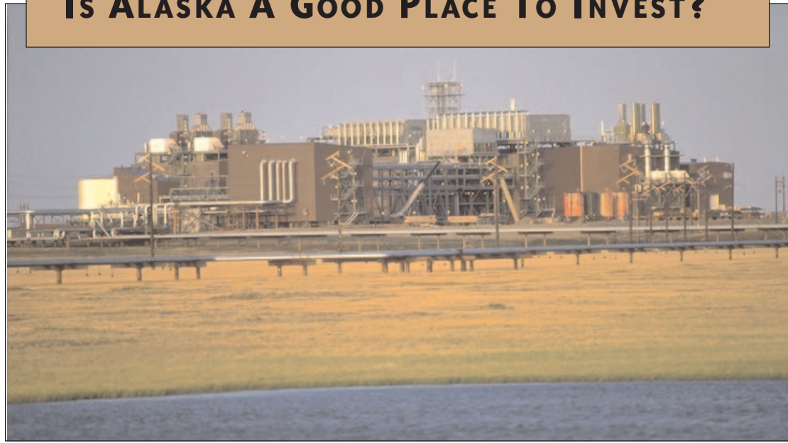
Alaska needs to attract a massive infusion of industry investment over the next ten years to prevent a sharp drop in North Slope oil production. Above is the Central Processing Facility at Kuparuk, the nation's second largest oil field. (ConocoPhillips Photo)
