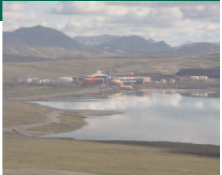
The Red Dog Mine dispute arose four years ago when TeckCominco Alaska applied to the State for a new diesel power generator permit. The mine is the largest producer of zinc in the world.
