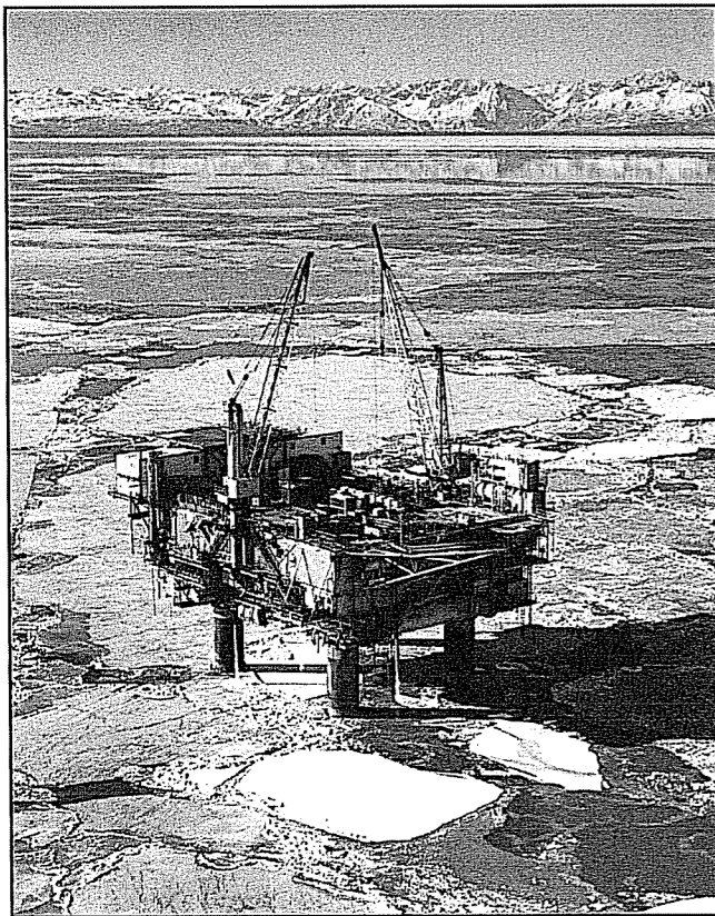
Existing infrastructure in the Cook Inlet region makes the area more attractive for investment by new, independent oil and gas operators. Pictured above is the Anna platform.
