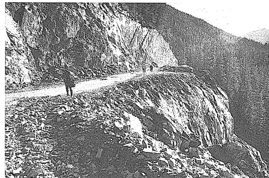
The access and bulk sampling road from tidewater to the U.S. Borax Quartz Hill molybdenum deposit was one of the most heavily regulated and monitored road construction projects ever undertaken in Alaska. Environmental permits in 20 different categories from nine separate agencies were needed before the ten mile road was completed in 1983.
