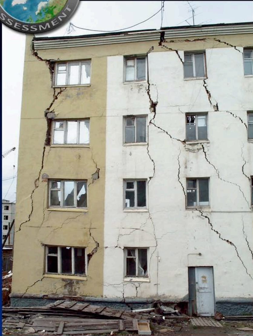
Thawing of permafrost is having a marked impact on buildings and ice roads
