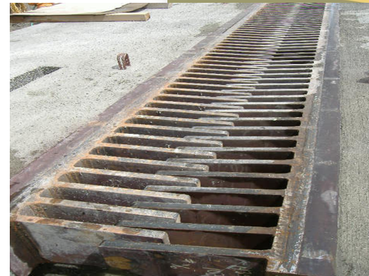
Nigliq Bridge Expansion Joint
