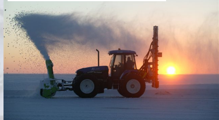
Ice Road Construction
