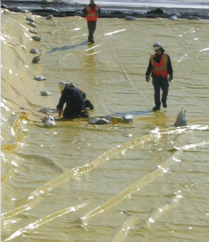
Drill Cuttings Storage Pit Construction - Apr '09
