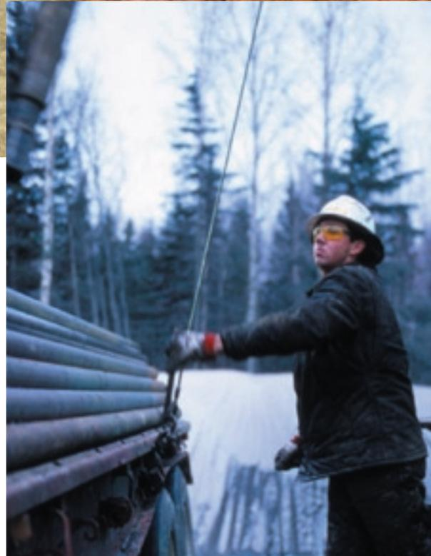
Under state law, CBM wells are engineered and built to protect all water. Up to three sets of steel well casing sealed with concrete from top to bottom ensure that water supplies are not contaminated, in accordance with state rules.
